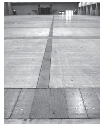
Pit and Sub-pit
